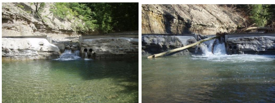
Figure 2c-3. Notching in the lower dam post-construction and pre-flood, and logs and rocks in notch after the Superstorm Sandy flood.
