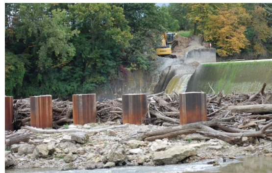
Figure 4: Notched Ballville Dam, Fremont Ohio
